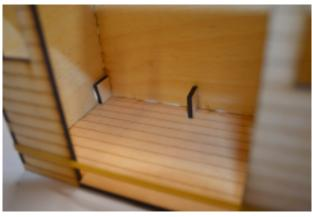
Glue the 3 seat supports to the floor and the back, one at each end and one in the middle, ensuring that the widest part is at the top.
